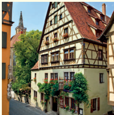
Stammhaus / Main Building
